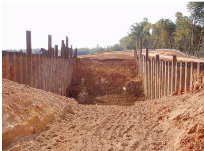
Figure 9 Excavation complete at 6.1m
