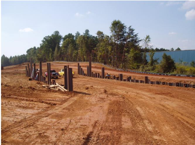
Figure 8 Installed sheet piles
